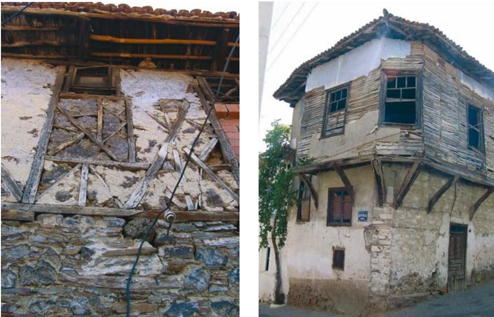
Fig. 6. Himis Technique (Kula) and Bagdadi technique (Bayindir) (right)
