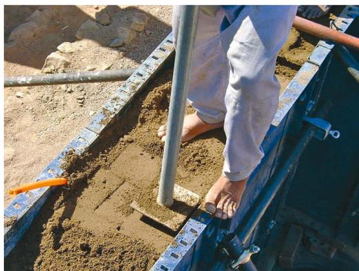
Fig.6. Rammed earth technique
