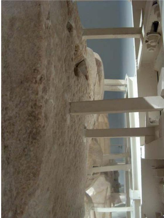
**Fig. 4.:** Iron bars used to keep the fragments in position. This arrangement close to the wall prevented the scanning of the rear sides of the figures. (Photo: author)
